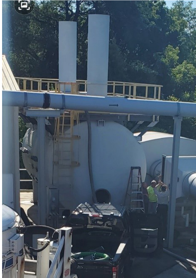
The odor control vessel is designed to hold 390 cubic feet of carbon media.
