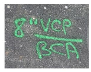
The sample picture illustrates marking most often used in Conshohocken. The number indicates the diameter of the pipe below, which in Conshohocken, ranges from 6" to 30." The top letters indicate what material the pipe is made from. VCP stands for Vitrified Clay Pipe and is what most sewer mains in Conshohocken are made of. The bottom letters tell the digger who the utility belongs to. BCA is Borough of Conshohocken Authority.
